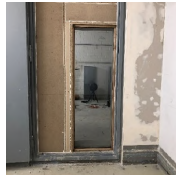
Figure 1: A double-shell installation mask in lightweight construction.
