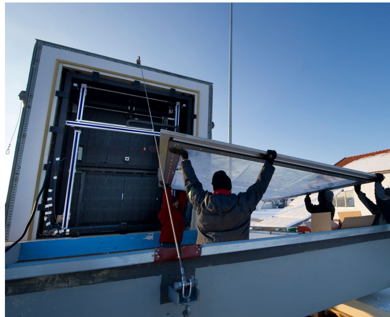
Installation of a multilayer membrane test specimen © Fraunhofer IBP
