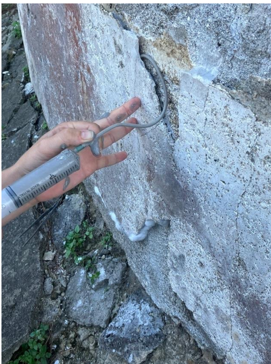
Figure 13 Grouting of the voids caused by the detachment of plaster layer (intonaco)
