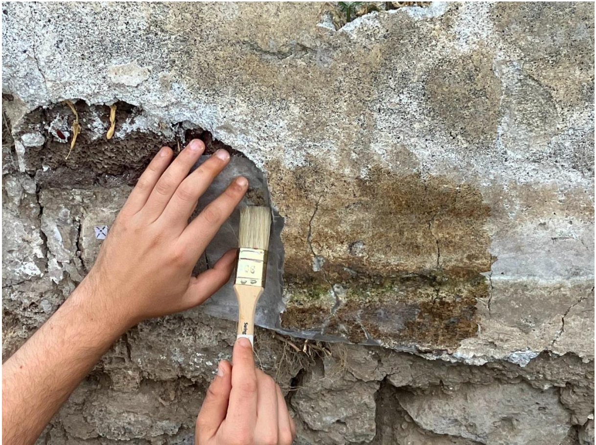
Figure 12 Application of a facing to temporary secure plaster using Japanese paper and carboxymethylcellulose
