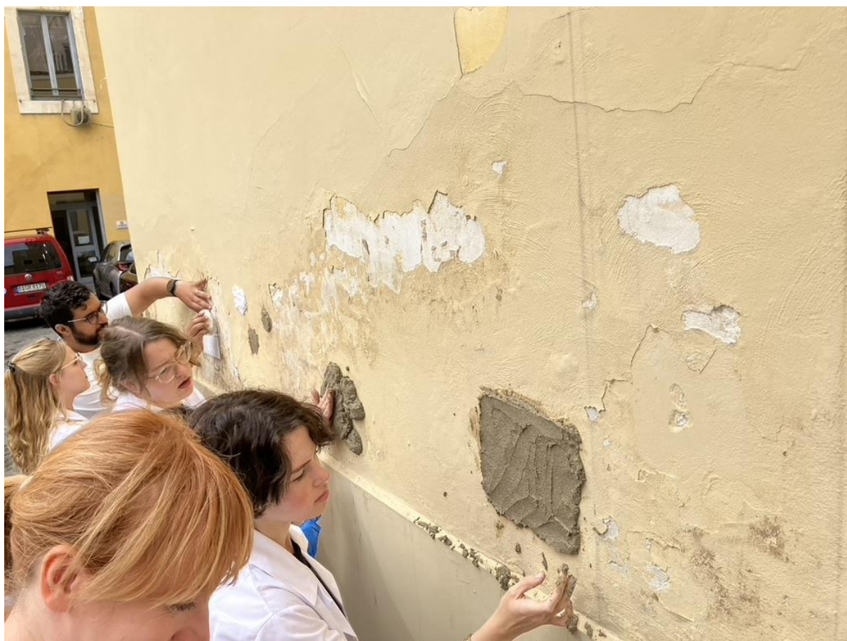
Figure 4 Participants applying salt-reducing poultices in the courtyard of ICCROM headquarters.
