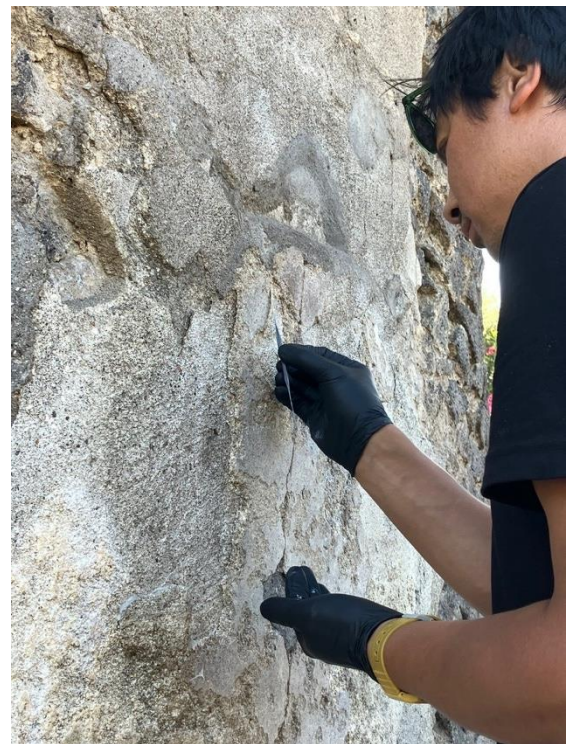
Figure 14 Application of restoration mortar to close open edges caused by the detachment of plaster layer
