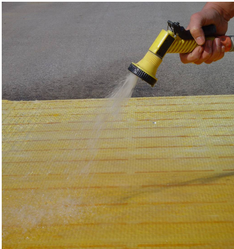
Figure 12: Spray-wetting of the glass fibre boards before installation.
