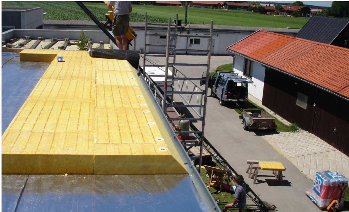
Figure 7: Laying of the wet insulation boards on the vapour barrier.
